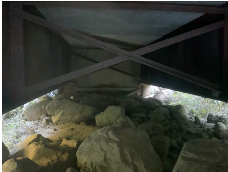
Left Bank Abutment when facing downstream
