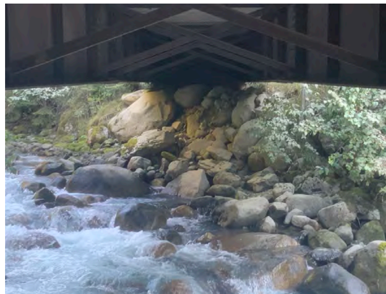
Left Bank Abutment when facing downstream
