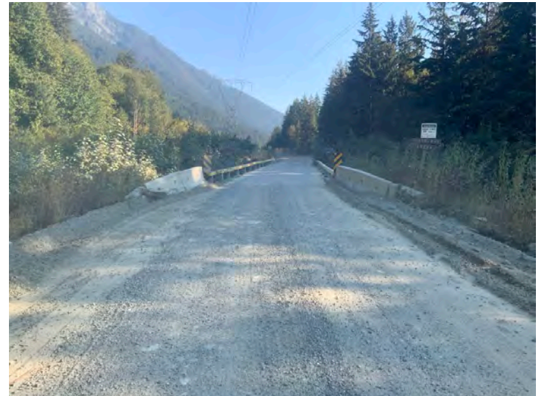
Approach from Right Bank when facing downstream
