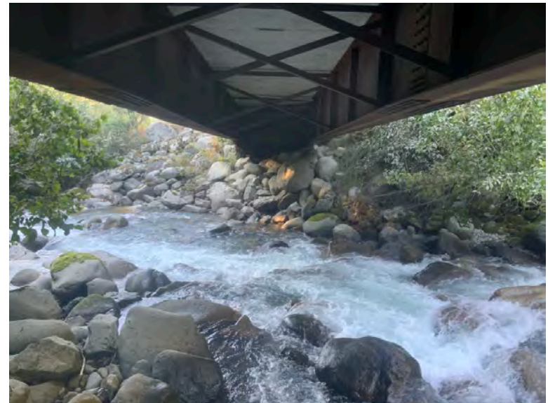
Right Bank Abutment when facing downstream
