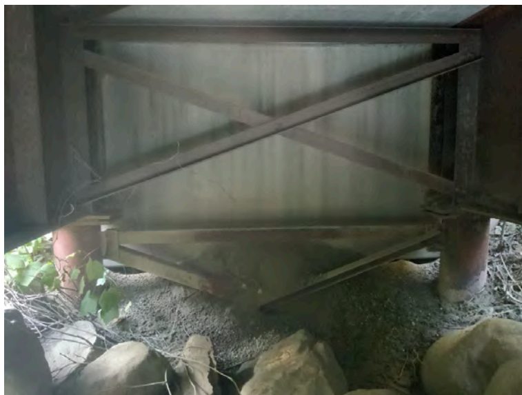
Right Bank Abutment when facing downstream
